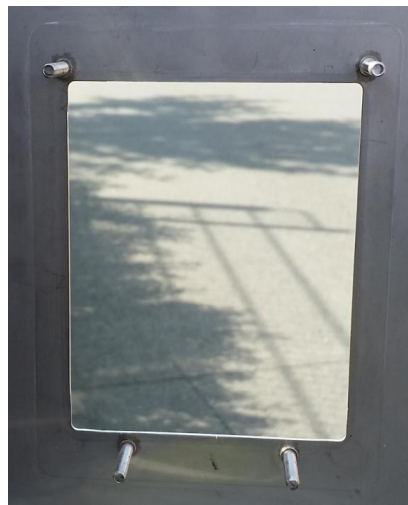
Fig. 4 Picture of front panel cutout for cVEND box with 4 threaded bolts
